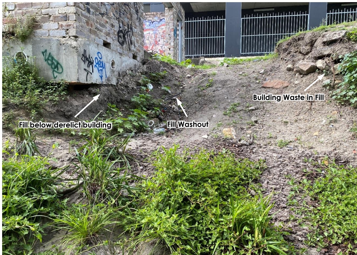
Figure 6: Fill embankment adjacent to derelict building within site (17 November 2021).
