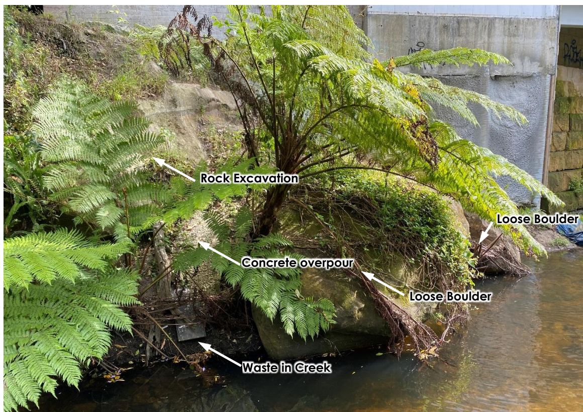
Figure 18: Northern Creek bank and embankment within site (17/11/2021).
