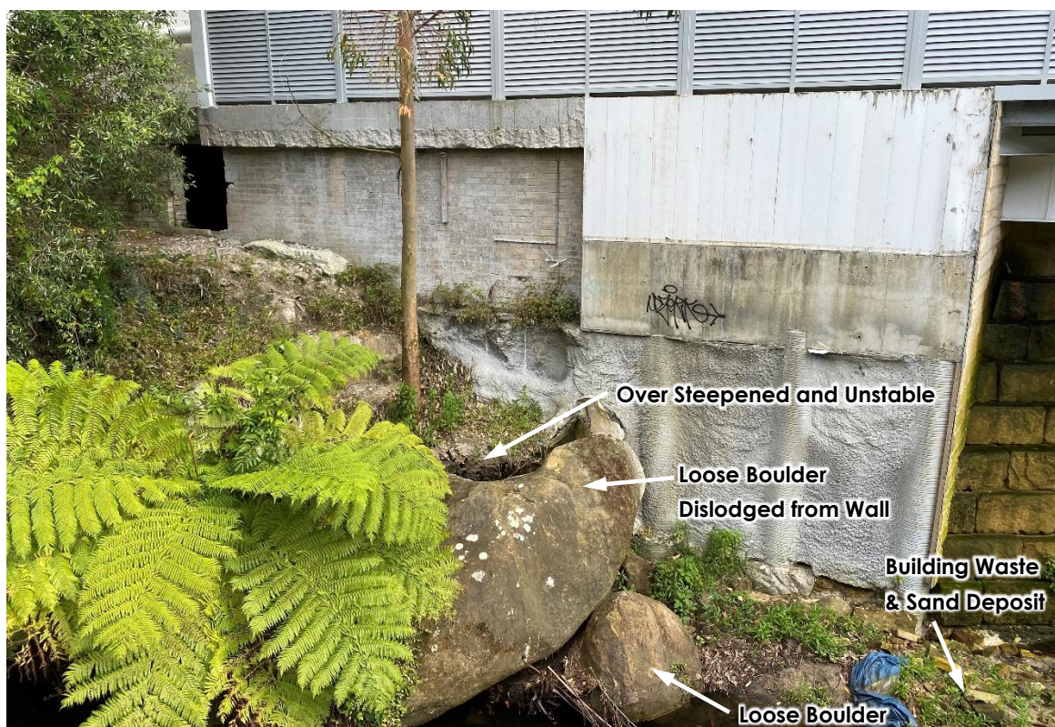
Figure 19: Northern Creek bank and embankment within site (17/11/2021).
