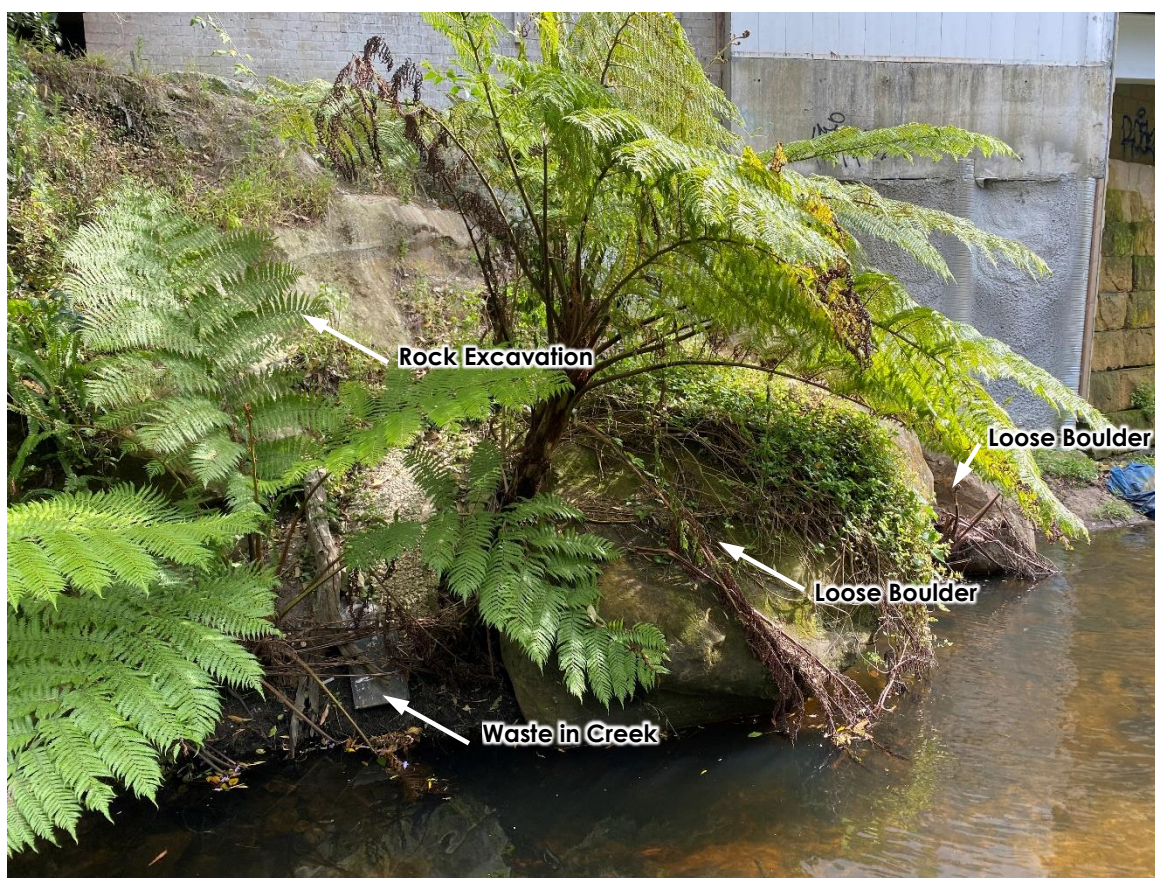
Figure 8: Northern Creek bank and embankment within site (17 November 2021).
