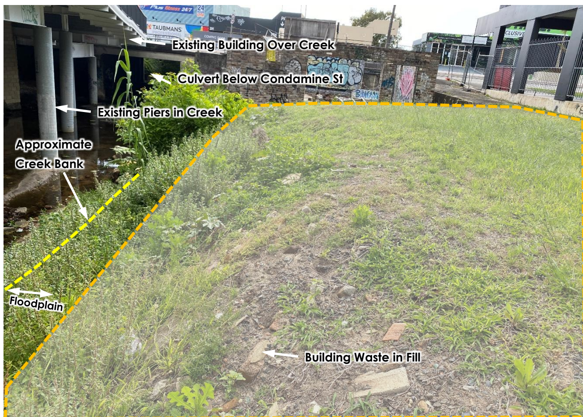
Figure 5: Fill embankment behind creek bank within site (17 November 2021).
